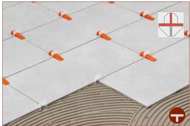
USE WITH "T" LAYOUT ON TILE INTERSECTIONS
